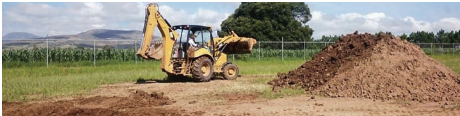
Constructing Activities in San Andrés Ixtlán, Mexico
